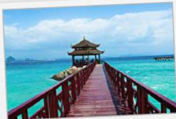
The trestle bridge in Wuzhizhou Island
